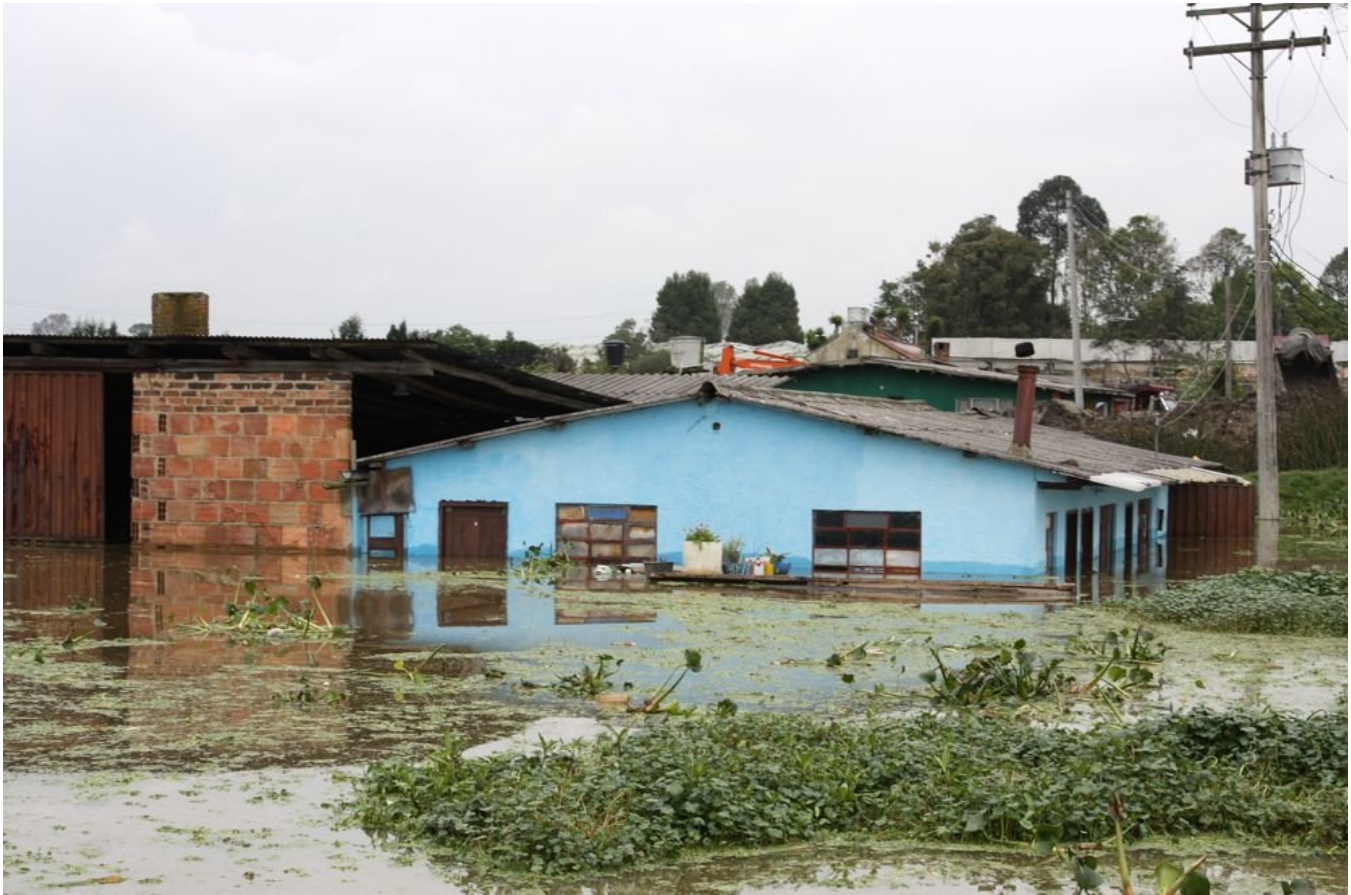
Flooded houses near Cota — in the Colombian department of Cundinamarca — are the result of unseasonably heavy rains in the Bogotá metropolitan area. [Richard McColl]
