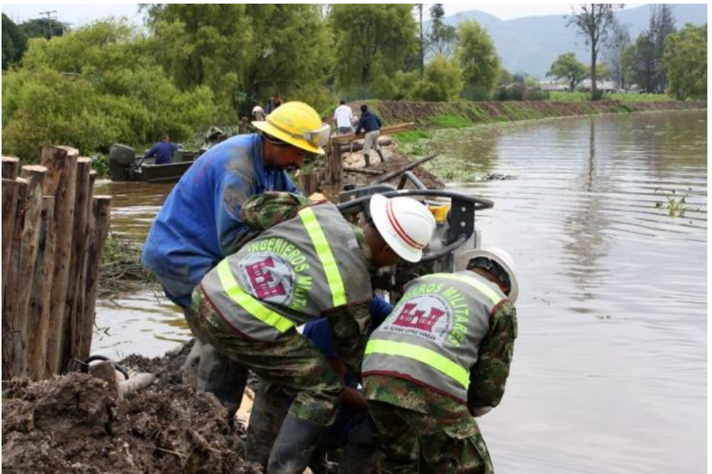
Colombian Army engineers work to erect barriers along the flooded banks of the Río Chicú near Bogotá. [Richard McColl]
