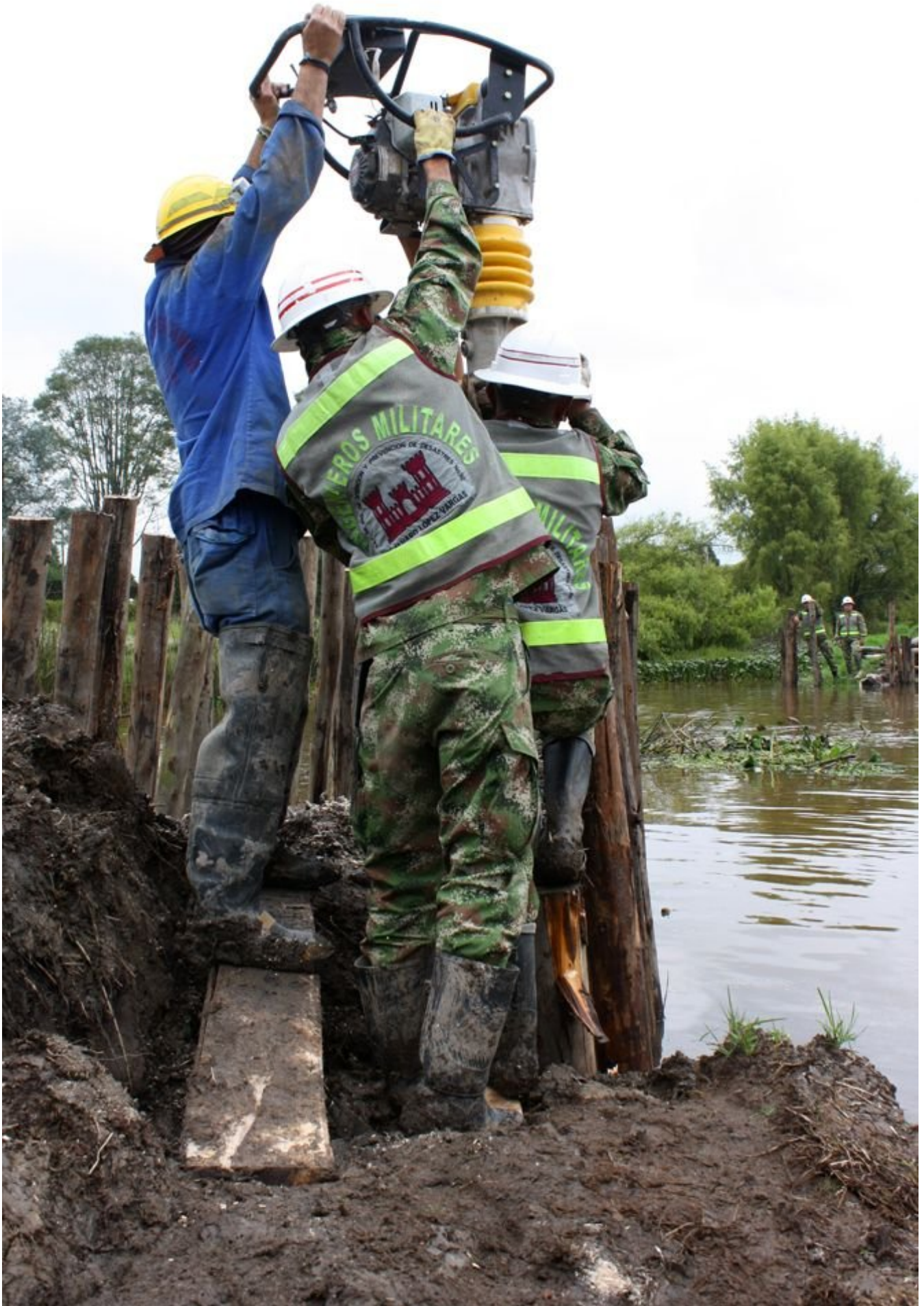
Colombian soldiers hammer in poles to stop flooding along the banks of the Chicú River near Bogotá. [Richard McColl]
